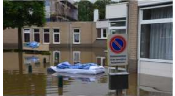
Figure 1. Flooding of an elderly home in Valkenburg aan de Geul in the summer of 2021 (source: R. Frissen, Sevagram).
